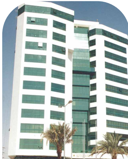
Federal Ministry of Finance Tower, Khartoum
